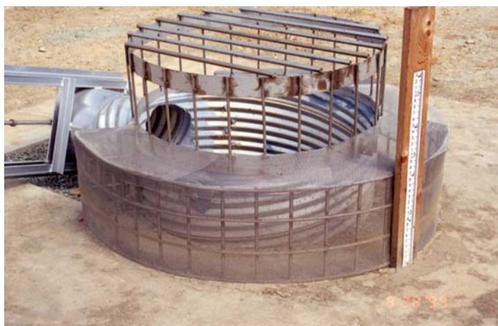
Figure 1 Example of Extended Detention Outlet Structure
