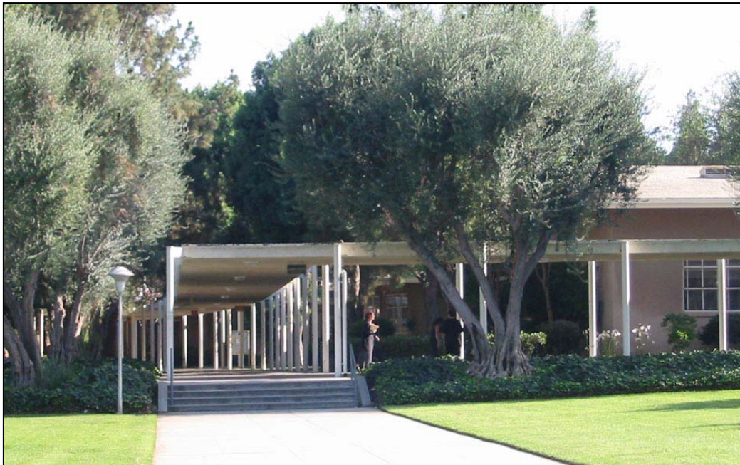
Figure 3-27: Administration Building and Covered Walkway
