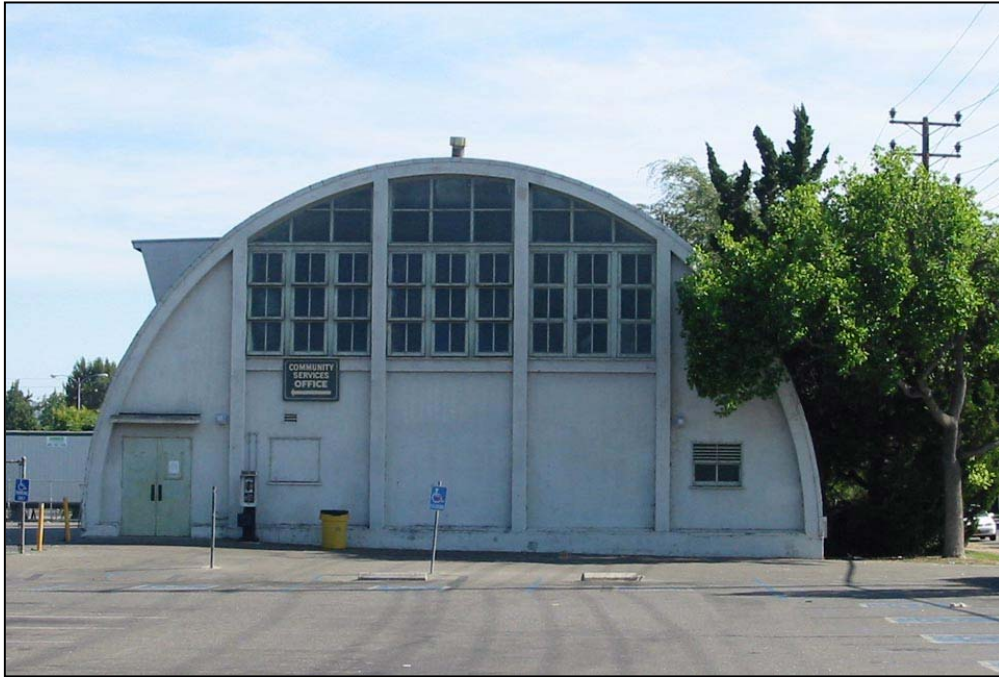
Figure 3-15: Field House (Original 1952 Gymnasium)
