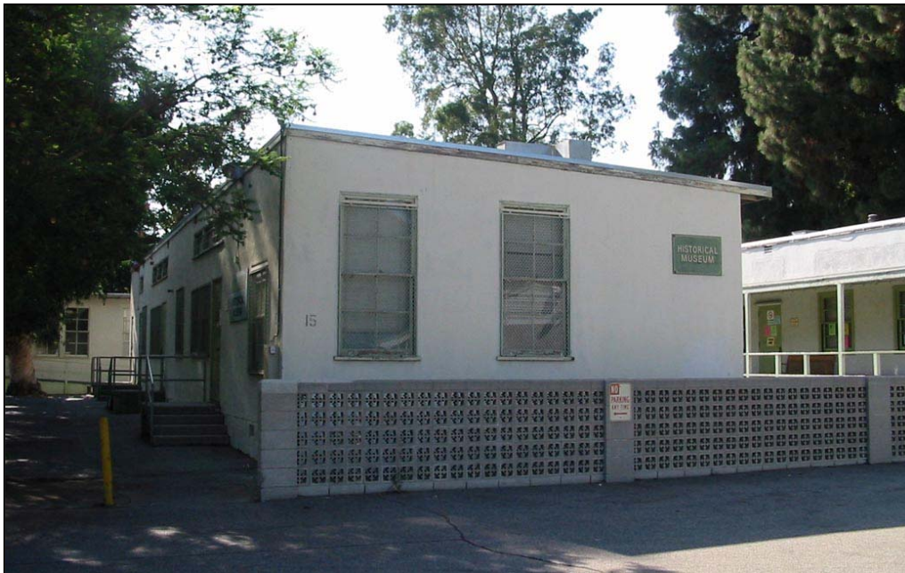
Figure 3-13: James Dodson Historical Museum Bungalow, View West
