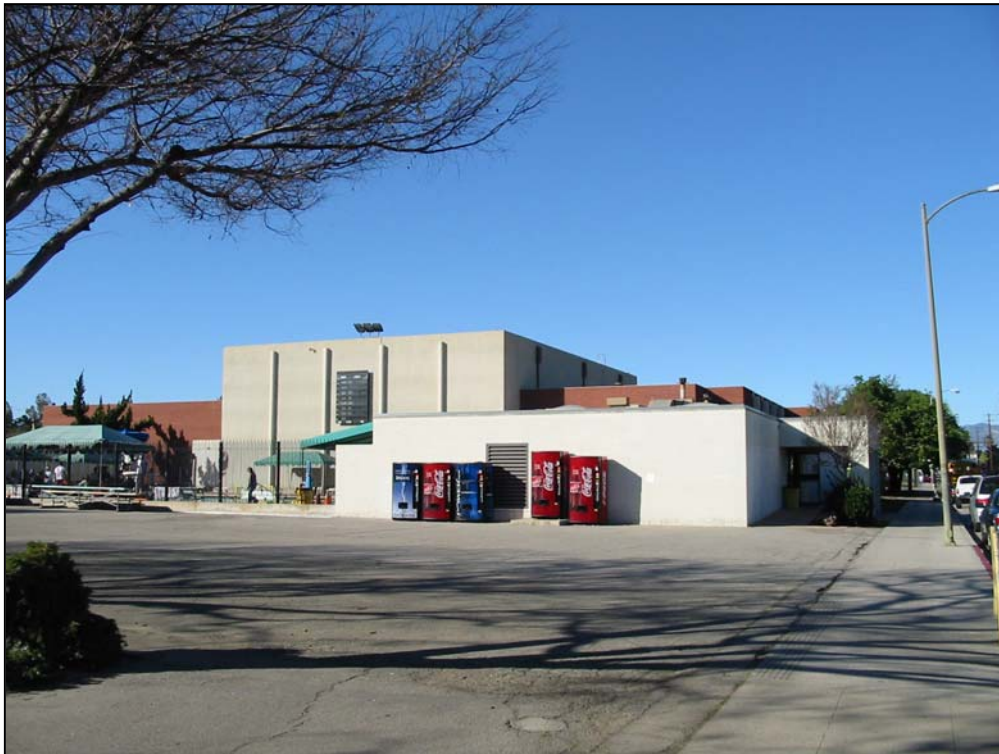
Figure 3-16: Paved Area Adjoining North Gym, Looking North
