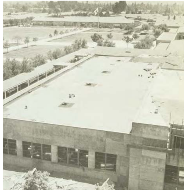
Figure A 1-3. The first library during its construction. This view shows trees of Monarch Square have been planted, circa 1960.
