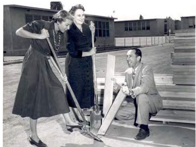
Figure A 2-2. Very little planting or shade around the bungalows, circa early 1950s.
